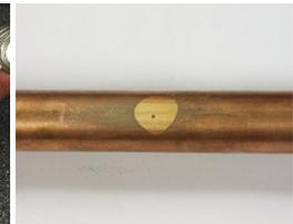
**6. Remove NSR Tab. Completed repair. Note resin covers an area larger than the actual hole.**
