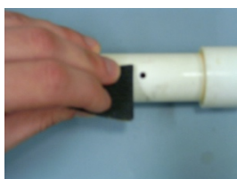
2. Clean/roughen area with 150 grit sandpaper.
