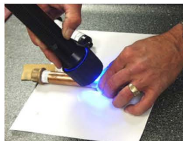
5. Shine NSR High Intensity Light directly on the applicator tab/resin for 30 seconds or until fully cured.
