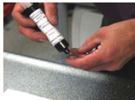
3. Cut Applicator Tab to desired size. Apply resin to NSR Tab.
