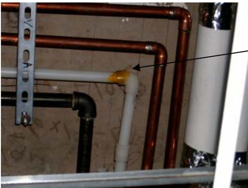
Repairs were done around joint. The joint was wet, but not under pressure.
