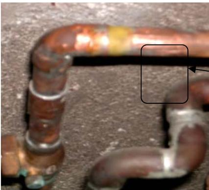
Copper pipe solder joint is repaired. Area that appears yellow is the resin. The area can be wet. The repair can be done at 28degF as well as at room temperature.
