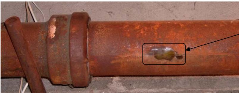
Repair to Cast Iron sewer discharge pipe. Resin can be applied in steps to cover larger areas.
