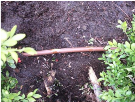
Pic 3. Repairs complete, pressure restored.
