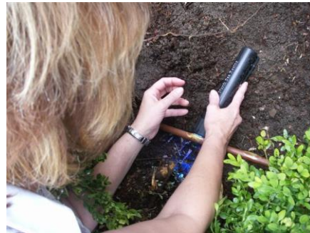
Pic 2.- With pressure relieved, immediate repair done despite moisture in line.
