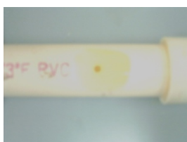
6. Remove NSR Tab. Completed repair. Note resin covers an area larger than the actual hole.
