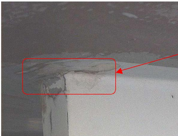
Picture 4. The Keel Stub developed cracks in the gelcoat protective layer. NSR resin was used to fill the cracks. Resin can be applied directly to the affected areas.
